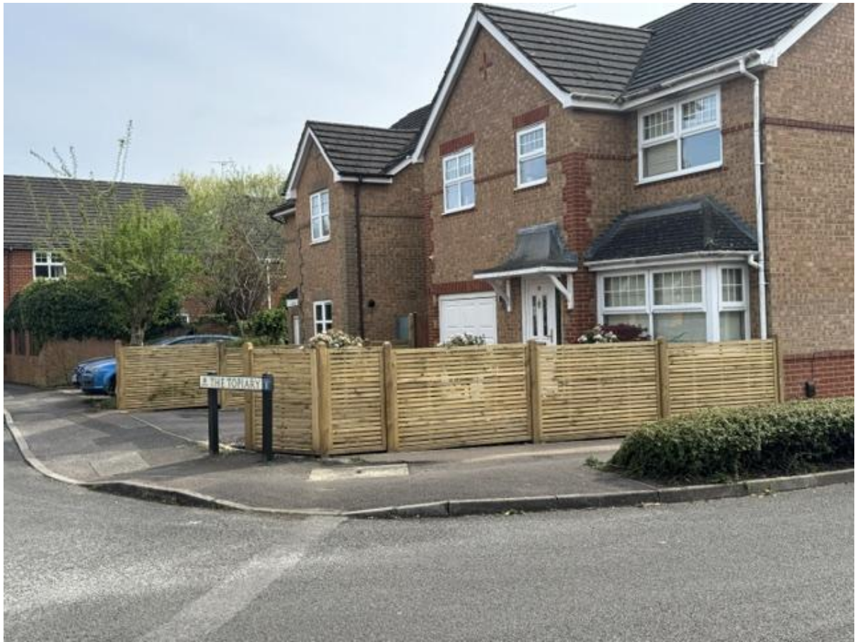
Figure 1 – view of fence at 28 The Topiary
